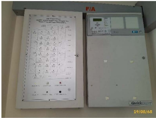
Fire Alarm Control Panel
